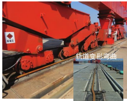
Fig 3. Container crane derailment caused by the bending of railway on gravity quay-wall
