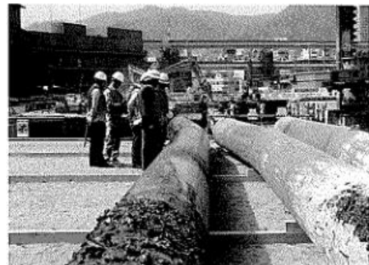
The damaged pile will be pulled out and inspected on site after the earthquake
